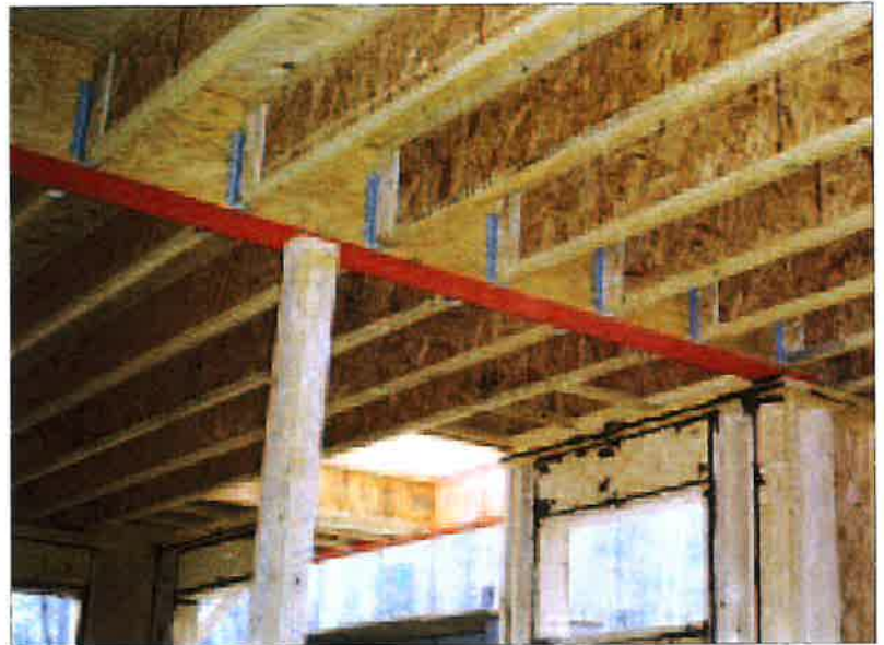
Figure 2. Floor joists laid flush with the top of engineered or steel beams will create a bump in the floor when they shrink (top drawing, left). In these situations, install the joists \frac{1}{2} inch high to accommodate the anticipated shrinkage (bottom drawing, left). Where I-joists meet an engineered lumber beam (above), you can install them flush since shrinkage is not an issue with I-joists.
