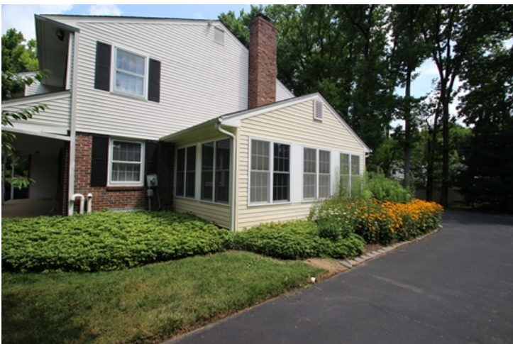
Sun Room Addition
