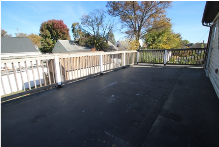
Roof Deck with access from Primary Bedroom
