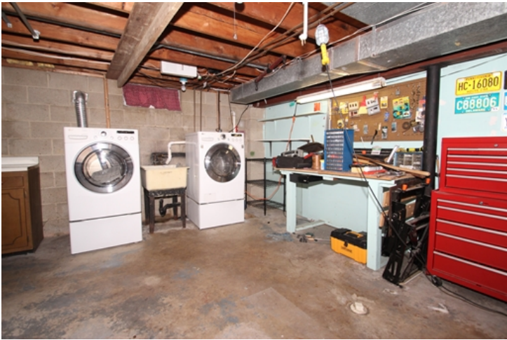
Laundry in Unfinished Area of the Basement
