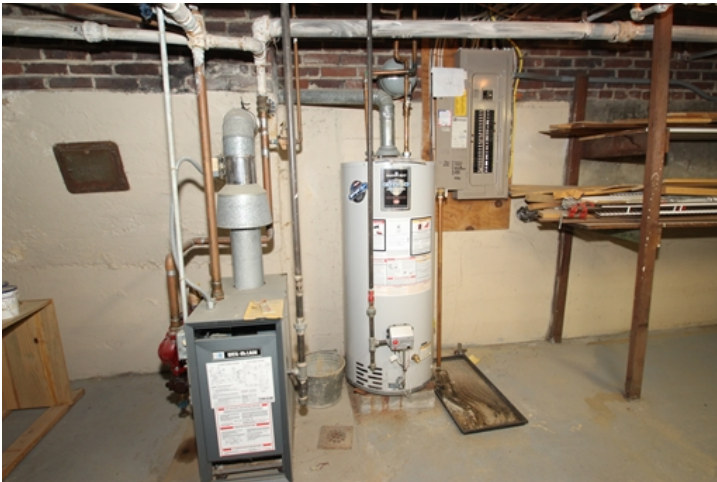
Utility area in basement
